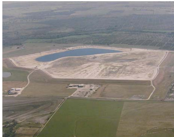
Figure 8: Conquista Project 245 acre Tailings Pond. Source: RRC
